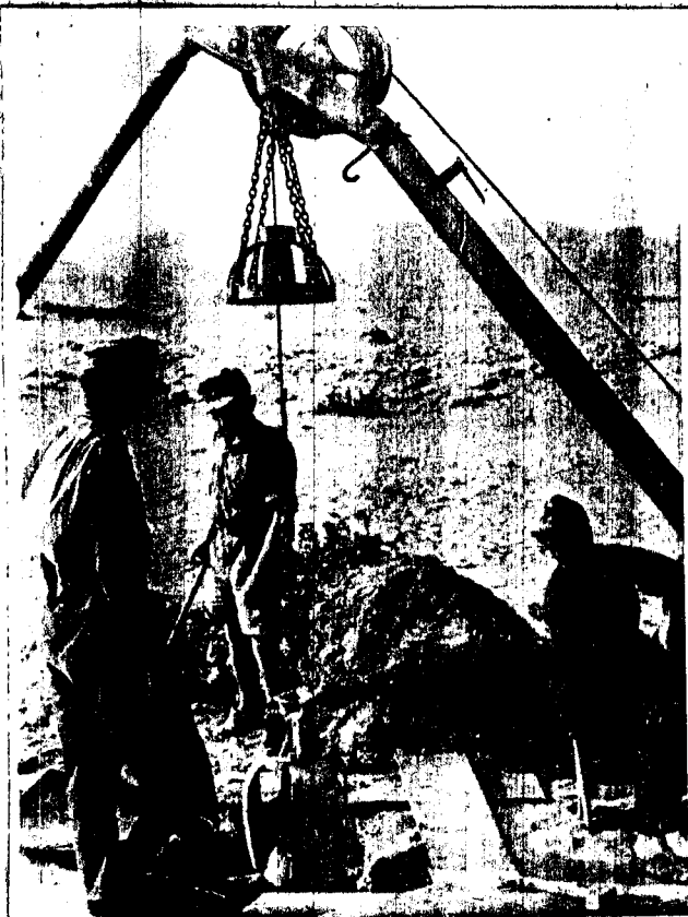
Right Remote Drilling Machine in Operation. Hammer in Drop
